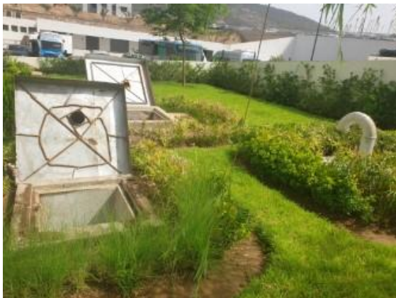
Water Conservation - Underground Water Reservoir (Fire and Sanitary and Cascade, Euromed University of Fez)
