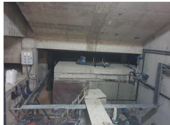
Water Conservation - Underground Water Reservoir (Fire and Sanitary and Cascade, Euromed University of Fez)
